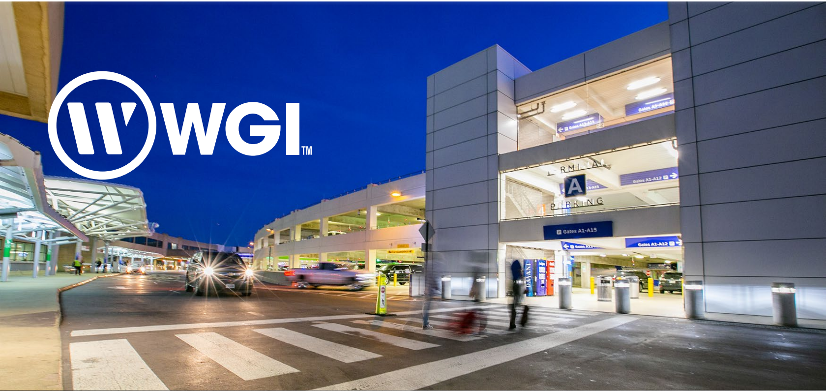
DALLAS FORT WORTH TERMINAL A AIRPORT PARKING STRUCTURE
