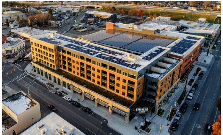
Three-level parking structure with a solar panel roof and wrapped on three sides by a grocery store, apartments above the grocery, office, and commercial.
