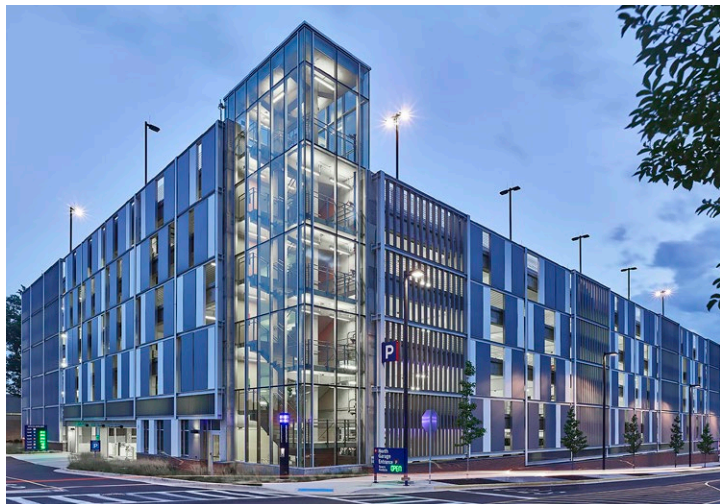
920 space university parking structure with an attractive and colorful aluminum panel and vertical louver facade that complements the Student Services Building. A real time level count parking guidance system helps users find an open space.
