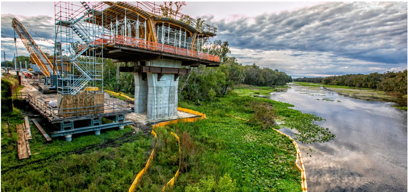
Wekiva Parkway, Segment 6 bridge construction, Orlando, FL
