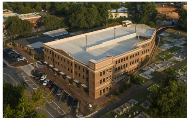
Four-level parking structure constructed entirely of precast concrete with integrally colored precast and face brick.
