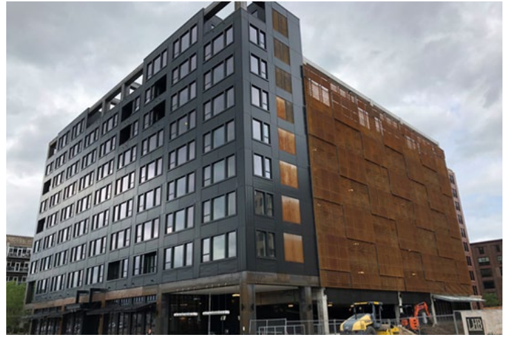
Eight-level, 400-space CIP PT parking structure. The development includes street-level retail, a nine-story residential building, and a 10-story office building.
