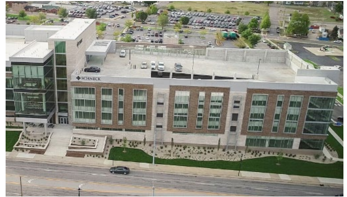
384-space parking structure with brick and stone façade that complements the main building on the medical campus. The project is part of a multi-year, multi-phase expansion which includes a five-story medical office. Additional surgical areas will also be developed with the main hospital to better serve patients.
