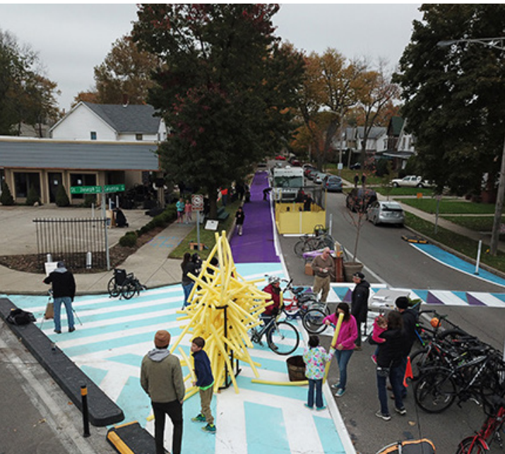
Quick Build projects like this one in Fort Wayne, Indiana support complete-street goals while enhancing business operations. Photo credit: Team Better Block and AARP
