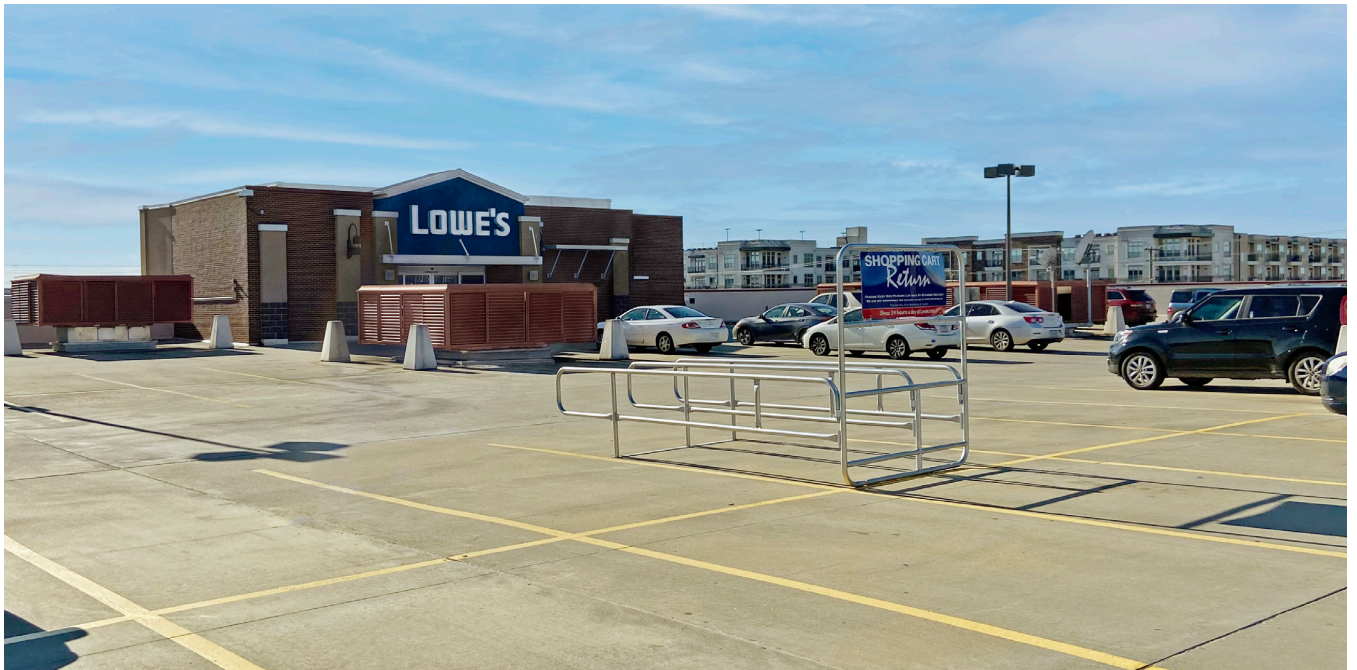
Store entrance from roof-top parking area, Charlotte, NC. Note the architectural treatment and protection of the roof-top HVAC units.
