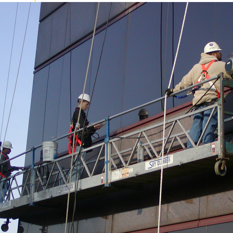
Curtainwall façade condition assessment
