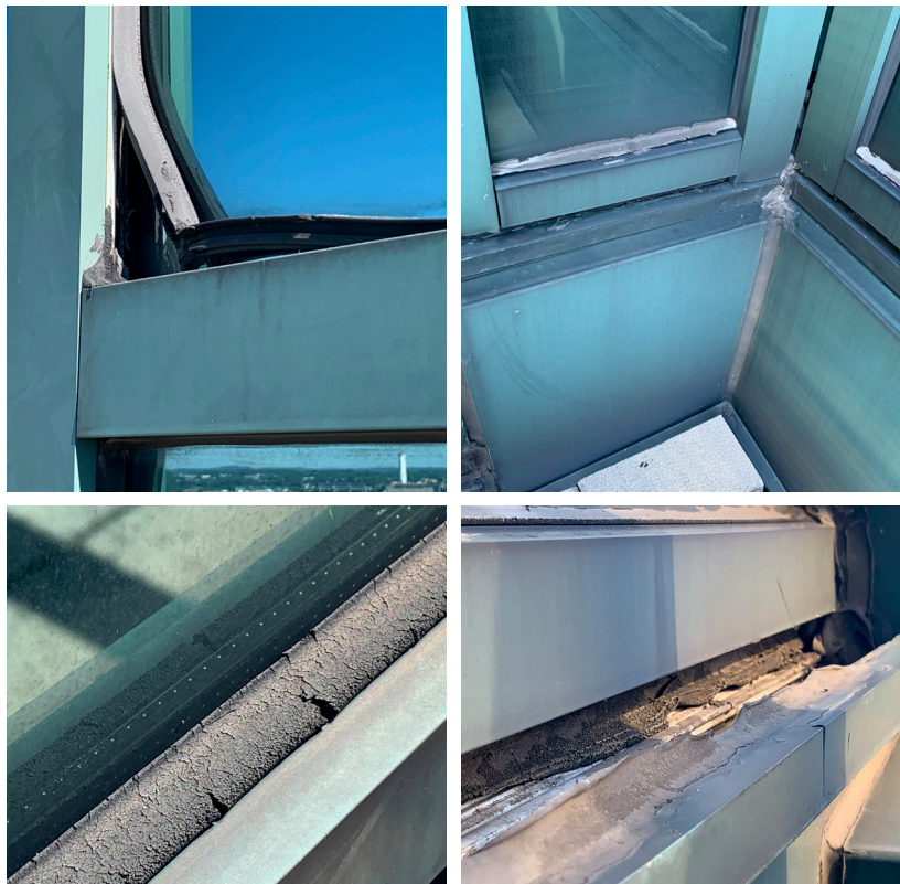
Curtainwall façade deteriorated conditions
