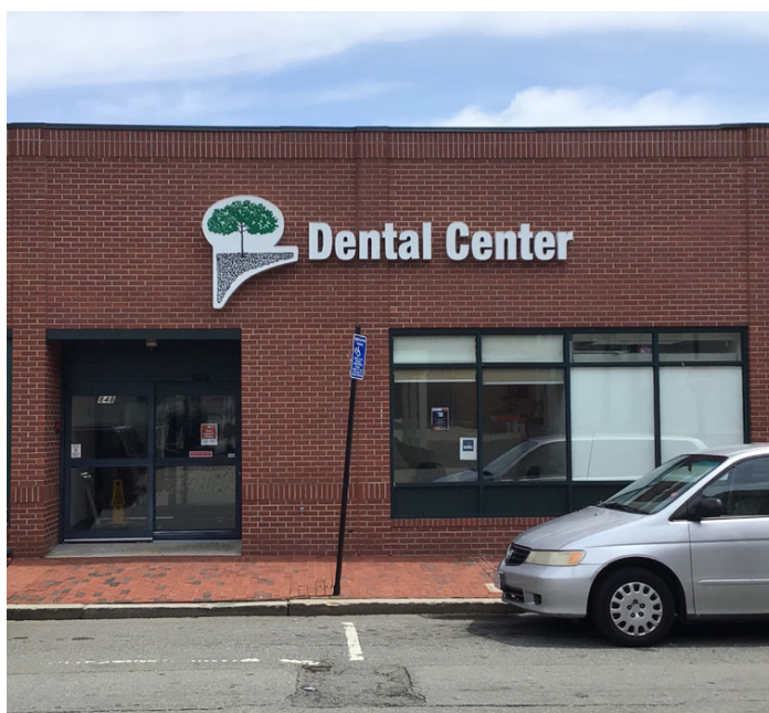
Example of Underutilized Storefront Source: WGI, May 2021
