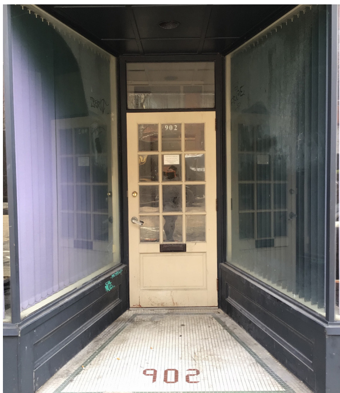
Example of Underutilized Storefront Source: WGI, May 2021
